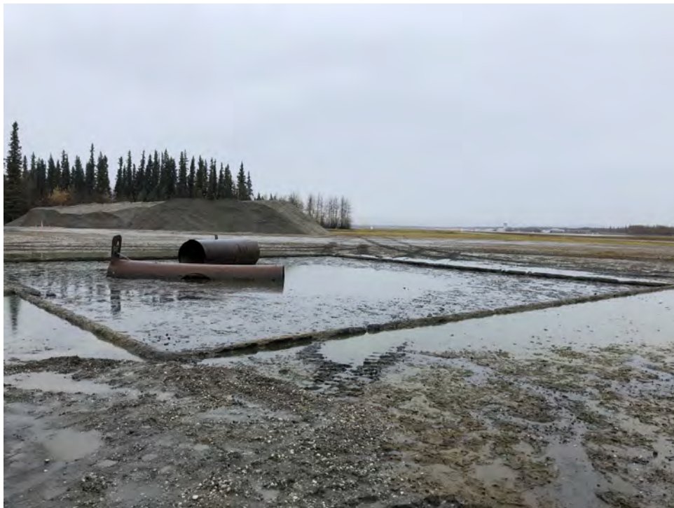
Photo 6: Partially Dewatered Fire Training Pit (September 29, 2019)
