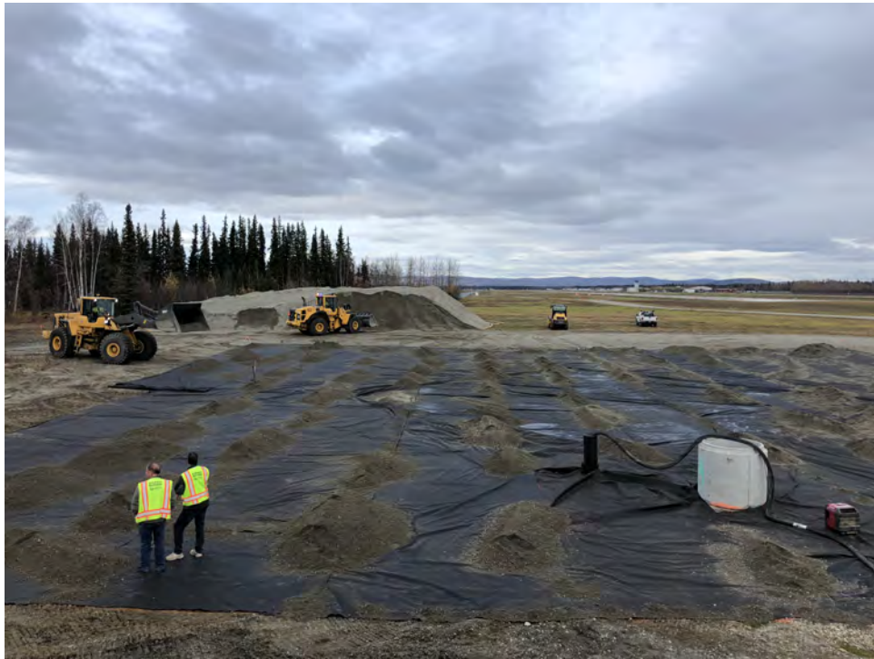
Photo 9: Geotextile Separation Fabric Placed (October 1, 2019)
