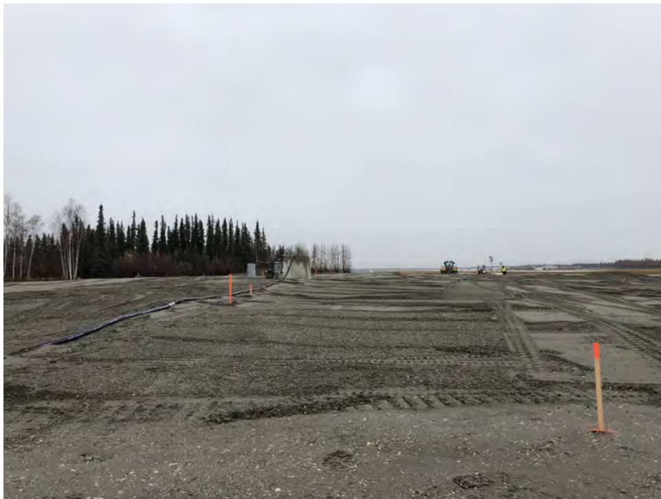
Photo 10: Placing Structural Fill (October 4, 2019)
