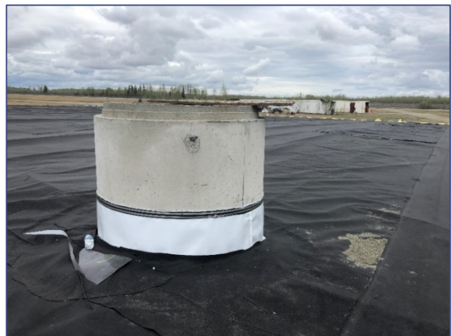
Exhibit 1-3: FTP sump extension (May 12, 2020)
