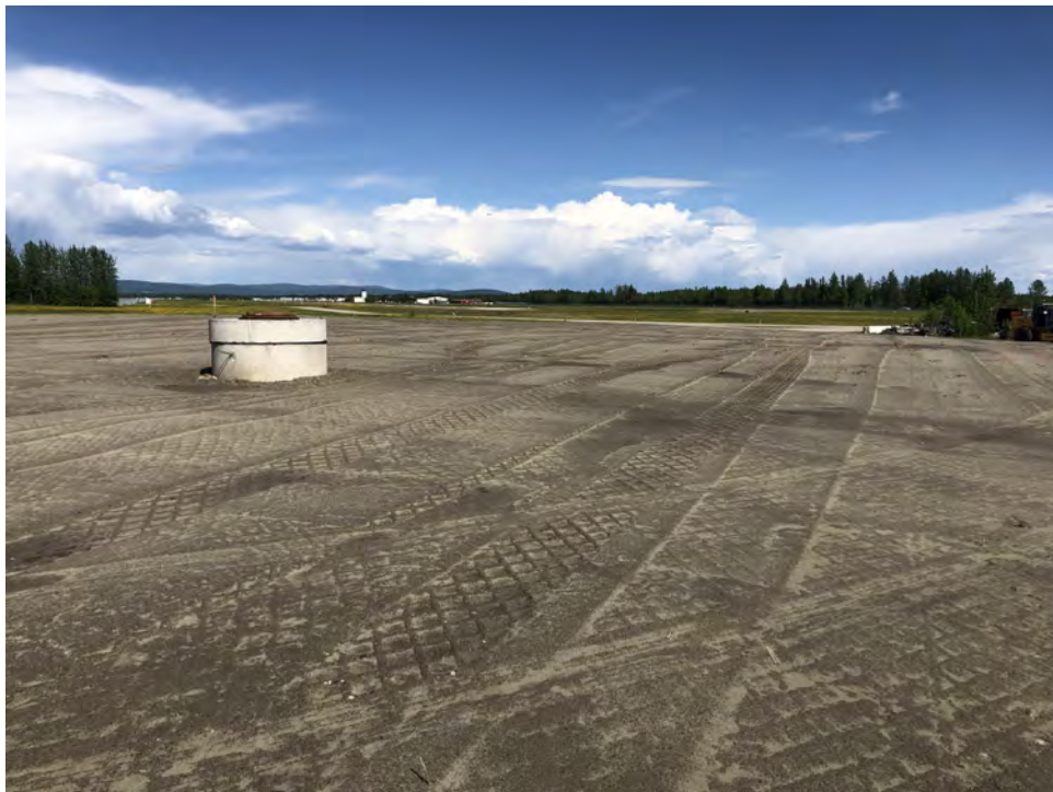
Photo 16: Silt and Topsoil Placed (June 5, 2020)
