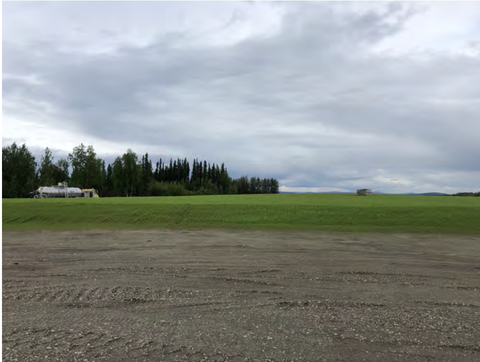
Photo 19: Watering the Cap Hydroseed (June 30, 2020)
