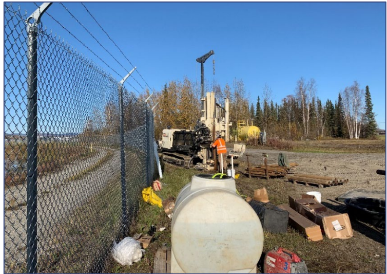
Exhibit 2-7: Installing MW-1901 well cluster (September 22, 2019)
