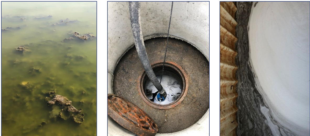
Exhibit 2-4: Pre-treatment FTP water Left: algae (September 10, 2019). Middle and right: foaming water (September 30, 2019).
