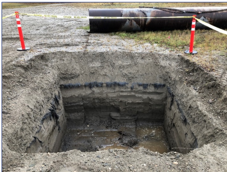
Exhibit 2-9: PFOS soil excavation outside FTP (September 19, 2019)
