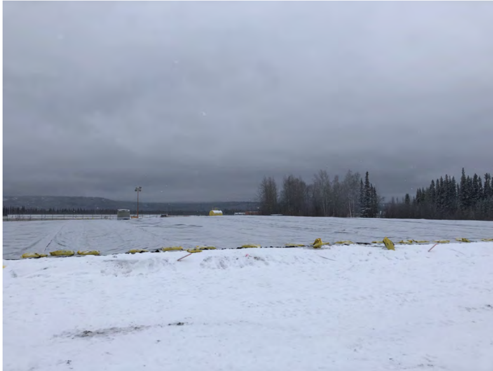
Photo 15: Geotextile and HDPE Geomembrane Liner Placed End of 2019 Construction (November 1, 2019)
