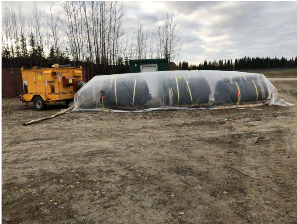
Photo 13: Heating the HDPE Geomembrane Liner in Preparation for Placement (October 22, 2019)
