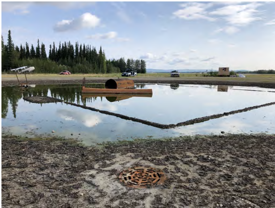
Photo 2: Fire Training Pit with Exposed Sump (July 19, 2019)
