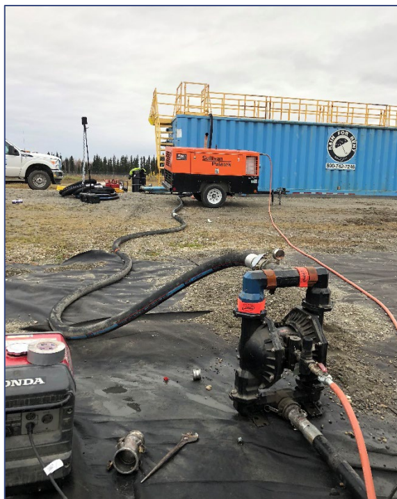
Exhibit 3-1: FTP dewatering (October 1, 2019)
