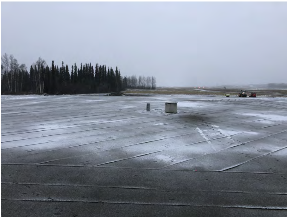
Photo 12: Structural Fill Placed, Ready for HDPE Geomembrane Liner (October 8, 2019)
