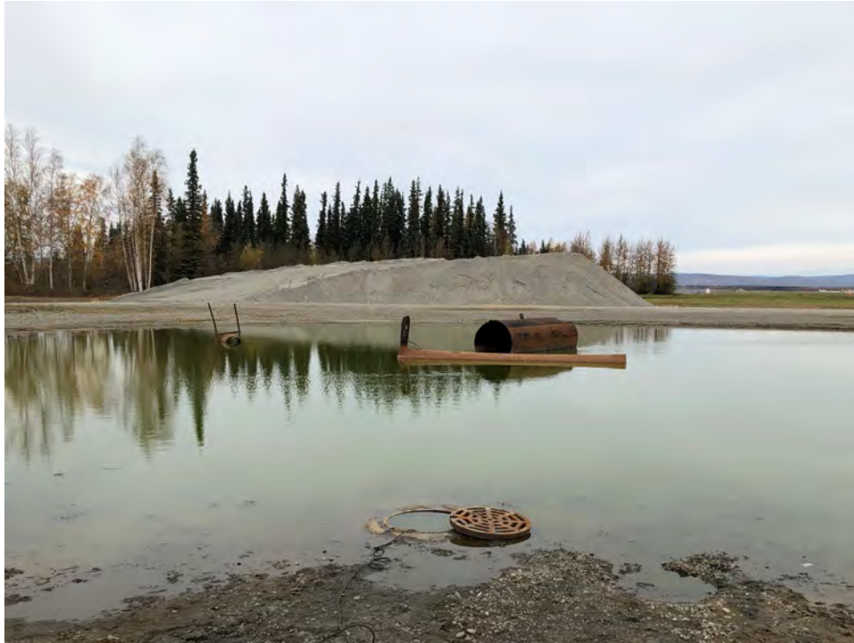
Photo 3: Fire Training Pit with Green, Algae-Rich Water (September 19, 2019)
