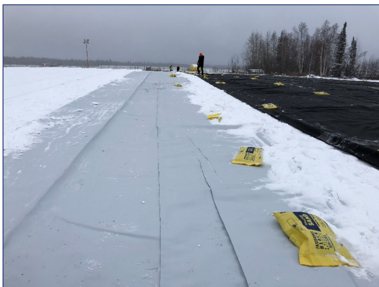
Exhibit 2-6: FTP geomembrane liner installation
