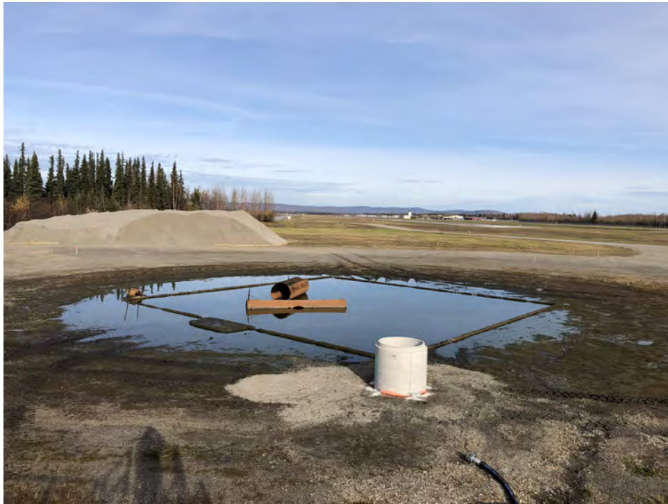
Photo 5: First Section of Sump Extension Placed (September 28, 2019)
