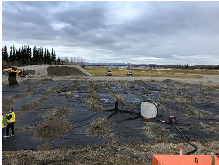
Photo 2: GNI and DOT&PF placing fabric rolls.
