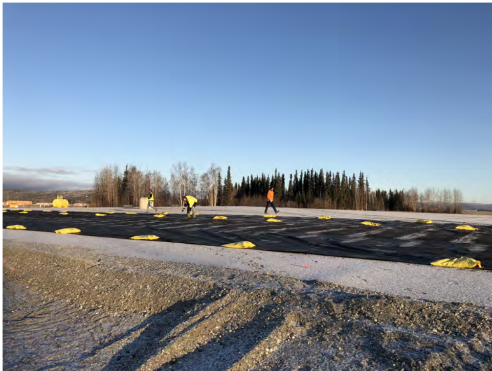
Photo 14: Placing Geotextile Separation Fabric and HDPE Geomembrane Liner (October 31, 2019)
