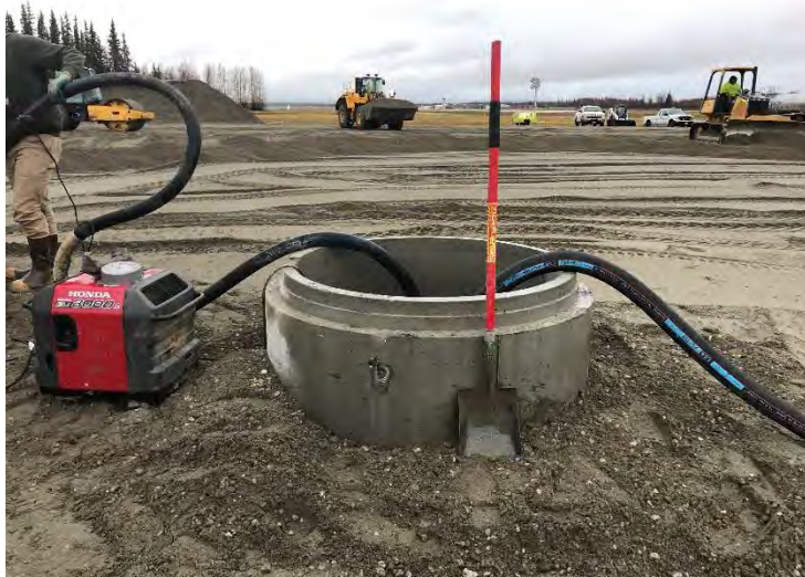
Photo 2: NRC pumping water from existing FTP sump.
