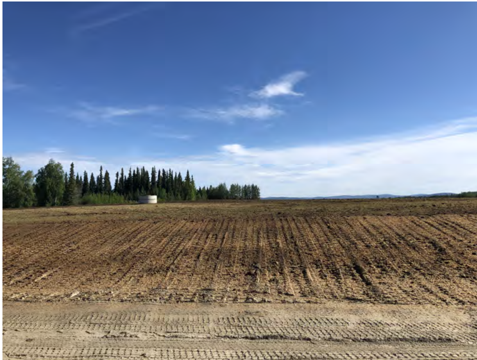
Photo 17: Hydroseed Placed, Cap Construction Complete (June 18, 2020)
