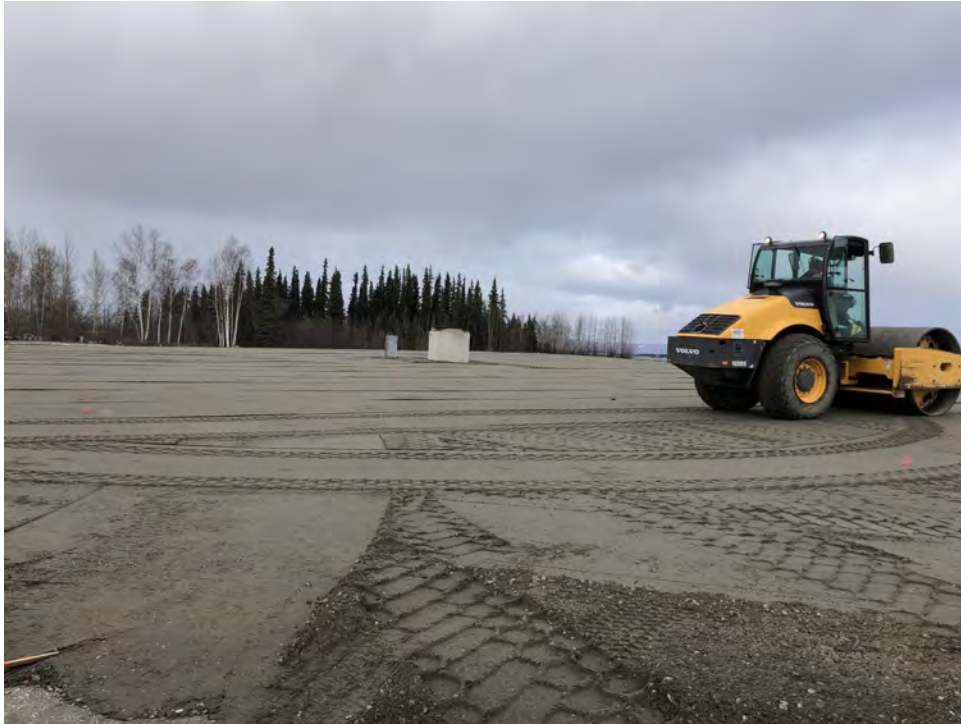
Photo 11: Compacting Gravel Fill (October 7, 2019)
