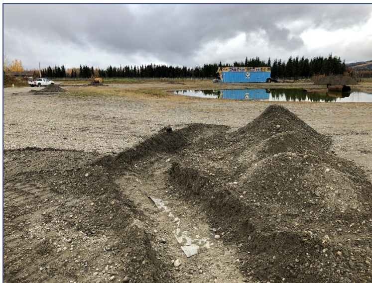
Exhibit 2-1: Locating the existing FTP liner (September 19, 2019)
