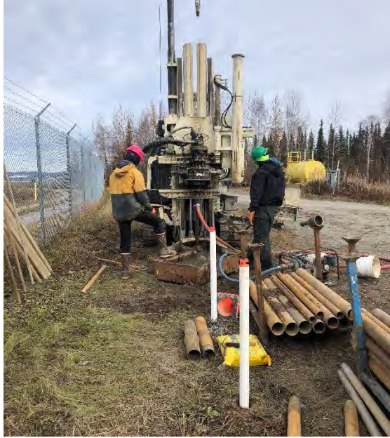
Photo 1: Drilling MW-1901-150, down-gradient from the FTP.
